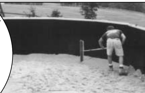
Build earth mound on top of wall guard using screened damp earth or pre-washed sand. Shape and compact earth mound to run 8" up from ground and 8" away from the wall. Do not use any material that will compress under pressure for the earth mound is an important part of the pool installation. It prevents the wall from lifting up and the liner from sneaking underneath the pool wall. Spread the remaining sand equally across the bottom of the pool. This will give you a 2" to 3" sand base.
